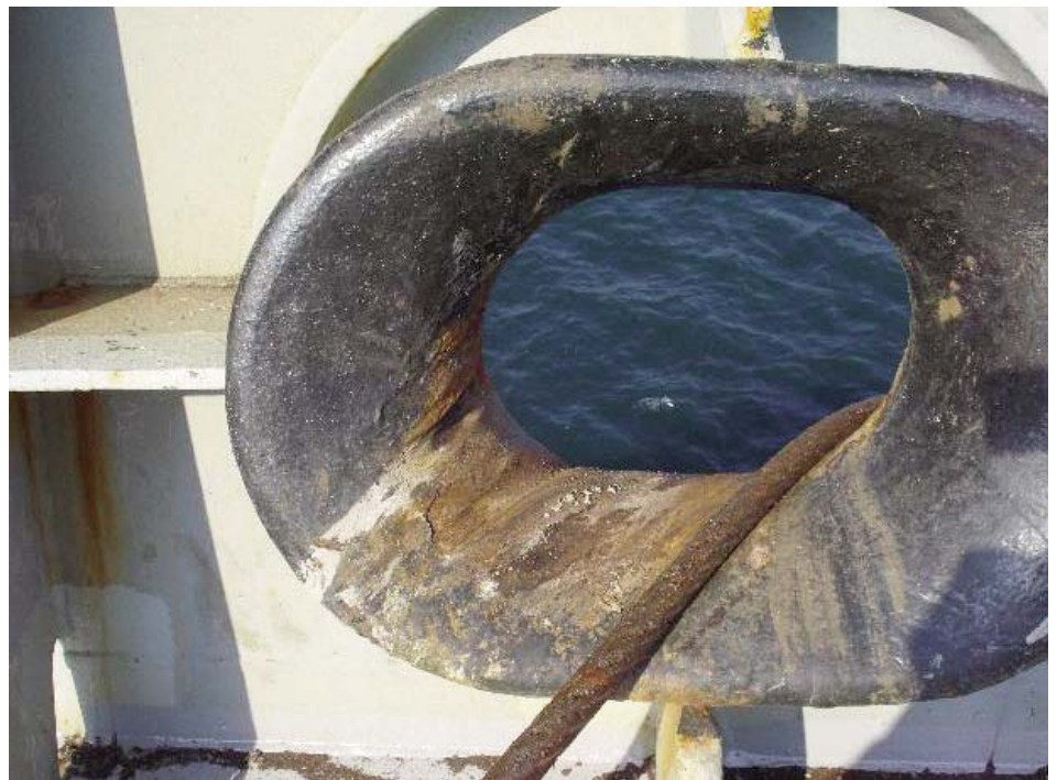
Closed chock and wire not properly greased.
